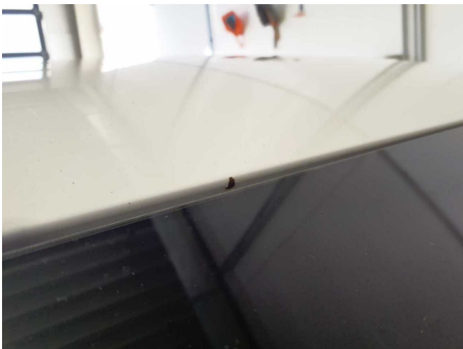
Damage 8: Roof: Roof - Corrosion - Repair and paint
