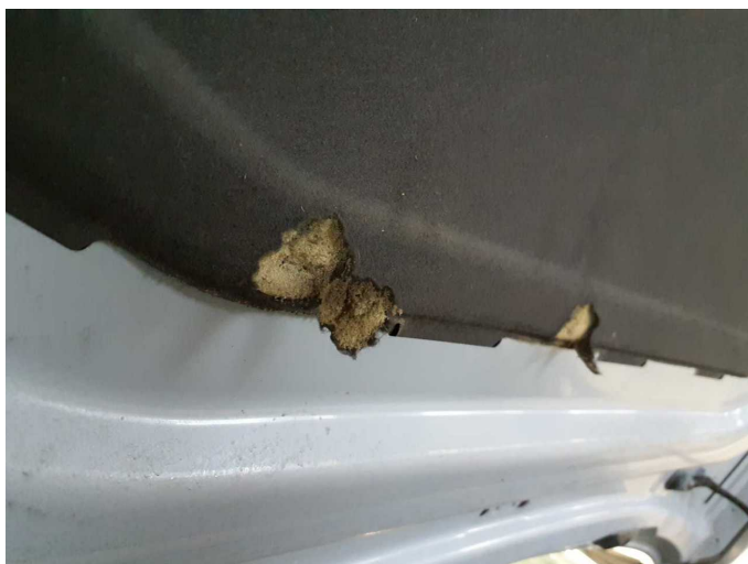
Damage 3: Bonnet: Insulation lining - Holes - Replace
