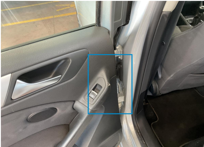
10. Panel Filling / Back Left Interior / Broken -
