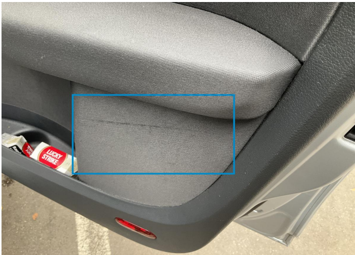
5. Panel Filling / Front Right Interior / Worn - out -
