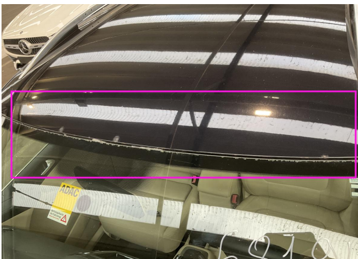
14. Roof Paint / Corrosion -
