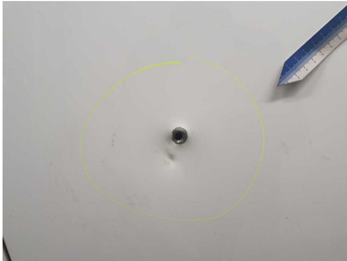
Damage 6: Sliding door, right: Sliding door - Holes - Repair and paint
