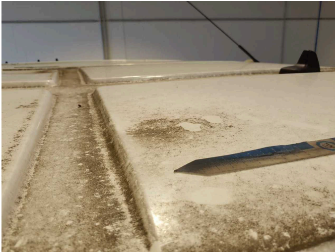
Damage 7: Roof: Roof - Corrosion - Repair and paint
