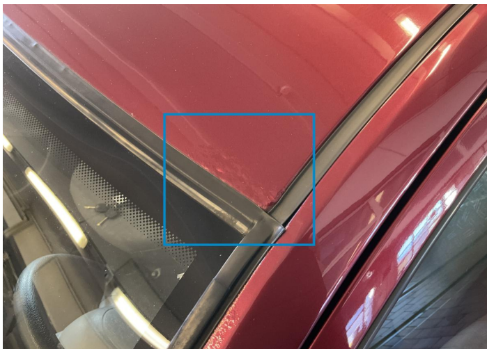
11. Roof Paint / Corrosion -
