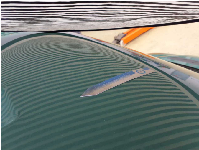
Damage 15: Roof: Roof - Deformed - Repair and paint
