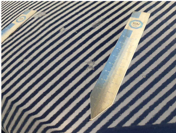
Damage 7: Roof: Roof - Corrosion - Repair and paint
