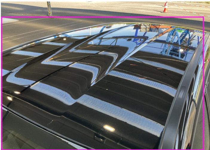
1. Roof Bodywork / Dent / Dent -
