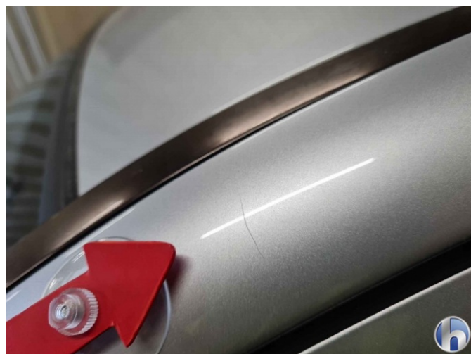
34. Roof frame - left
