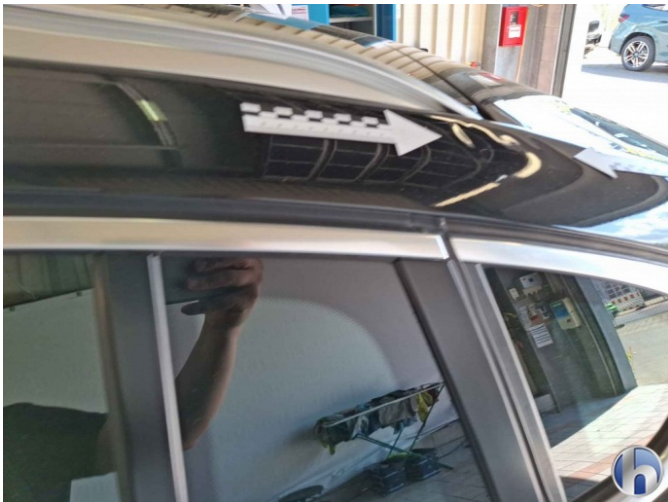
12. Roof frame - left
