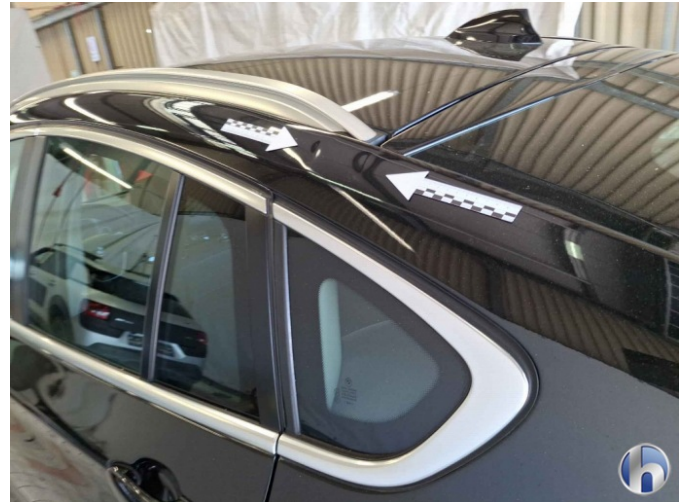
12. Roof frame - left
