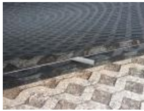
Door seal FR, Deformed / Strained, Repair/replace (lump sum)
