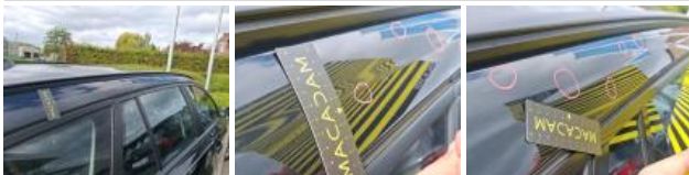
Roof pillar R, Hail damage, Repair and paint (complete)
