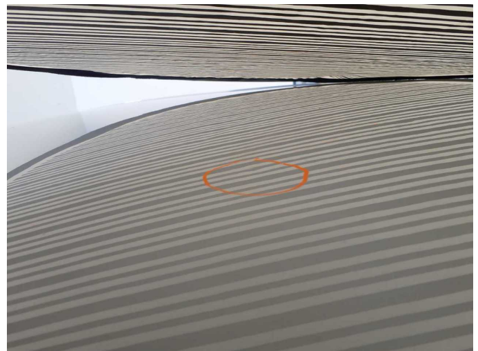
Damage 2: Roof: Roof - Damage by hail - Smooth repair work
