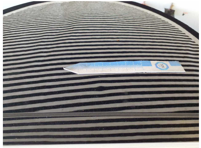
Damage 3: Roof: Roof - dent(s) - Smooth repair work
