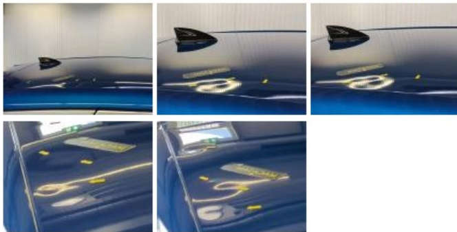
Roof, Dent(s), Repair and paint (complete)
