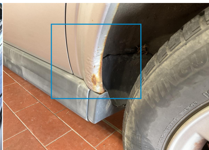
4. Side Panel / Back Left Paint / Corrosion -
