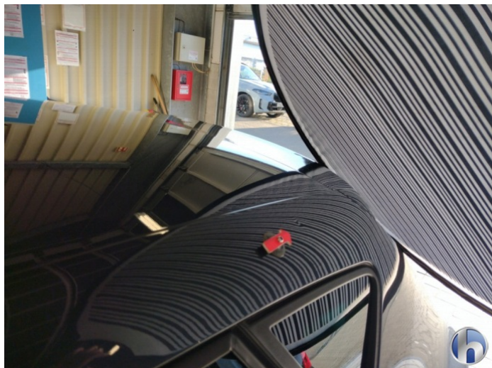
8. Roof frame - left
