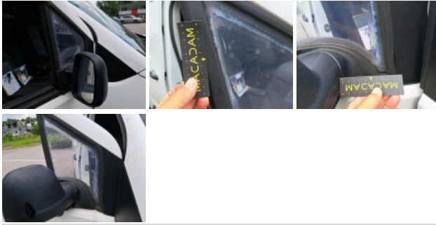
Outside rear-view mirror housing R, Broken, Replace
