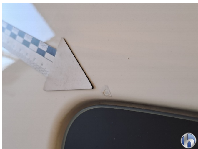
15. Roof frame - right
