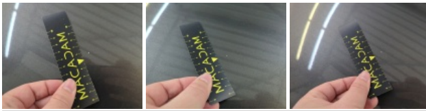
Bumper FM, Crack, Repair and paint (complete)
