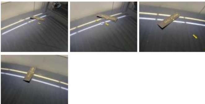
Roof, Dent(s), Paintless dent repair
