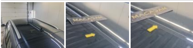
Roof, Dent(s), Repair and paint (complete)
