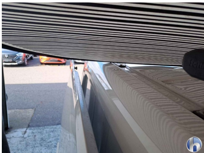
38. Roof frame - right
