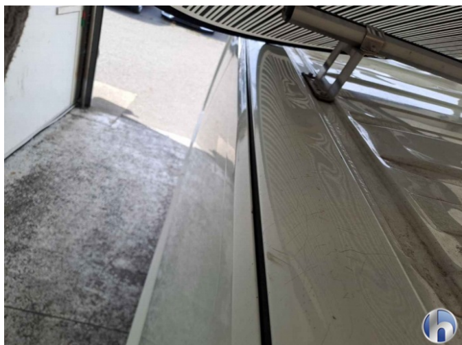
36. Roof frame - right
