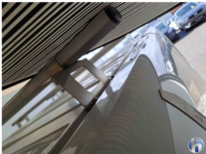
22. Roof frame - left
