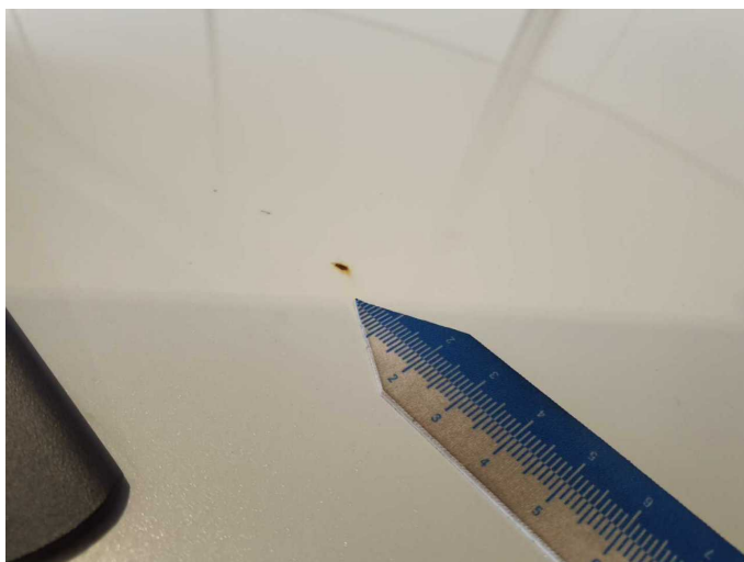
Damage 12: Roof: Roof - Corrosion - Repair and paint
