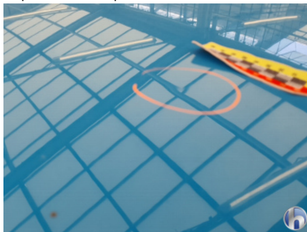
10. Roof 1 dent - Gentle refurbishing
