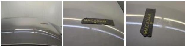
Roof, Chemical polution, Polish
